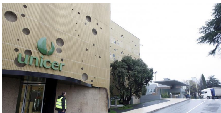
Super Bock Group | Matosinhos Elevators: 10
