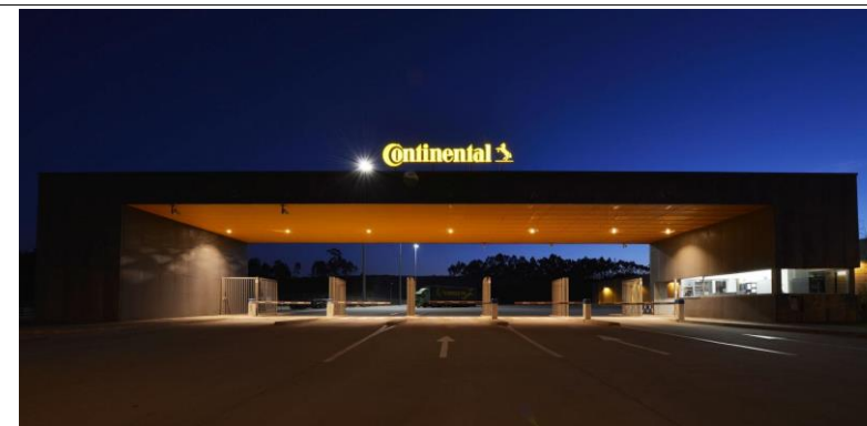
Continental | Lousado Elevators: 5
