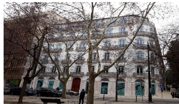
Liberdade 203 | Avenue Elevators: 7
