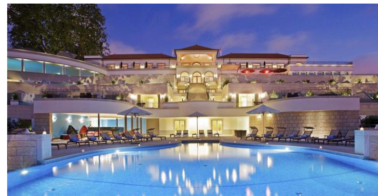
Yeatman Hotel | Vila Nova de Gaia Elevators: 17
