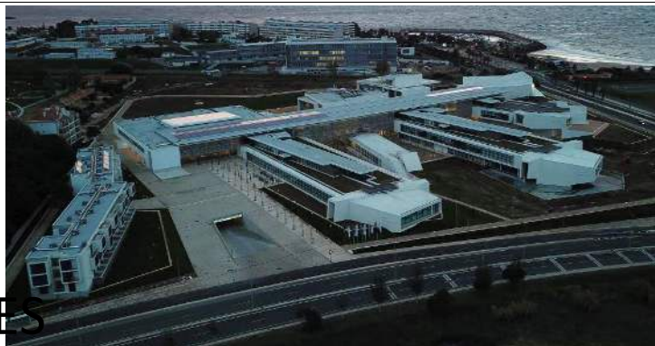
Nova School of Business & Economics | Oeiras Elevators: 12
