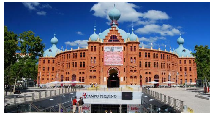
Campo Pequeno | Lisboa Elevators, escalators and autowalks: 33
