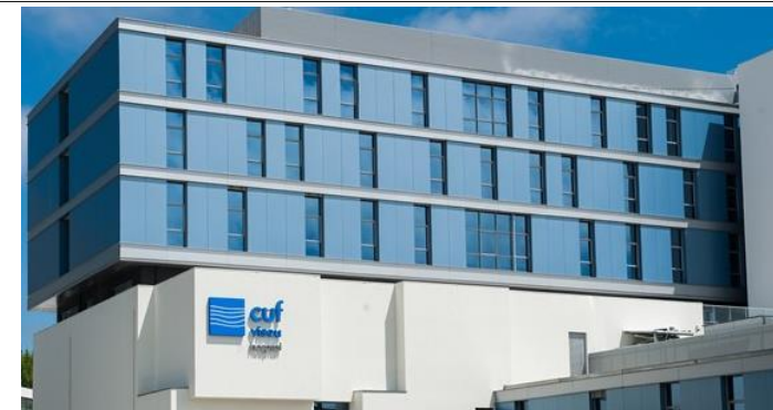
Hospital CUF Viseu Elevators: 7
