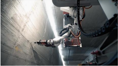
Schindler's R.I.S.E. Robotic Installation System for Elevators
